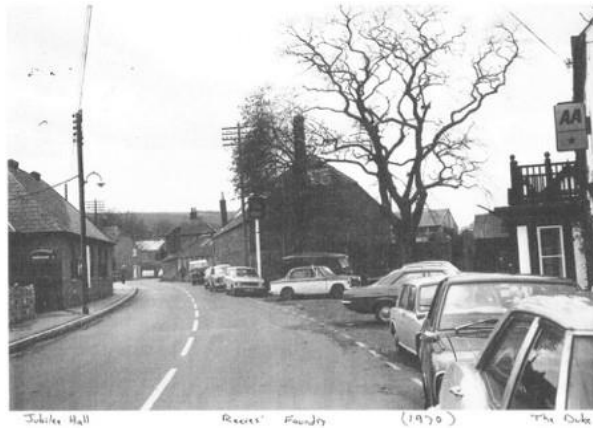
View west along the main road - 1970
