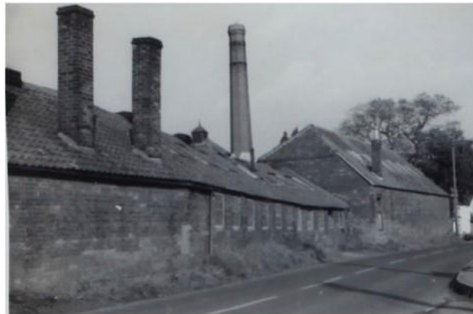
Smiths shop, fitting shop (with many windows), foundry and 'The Duke'. Boiler house chimney behind
