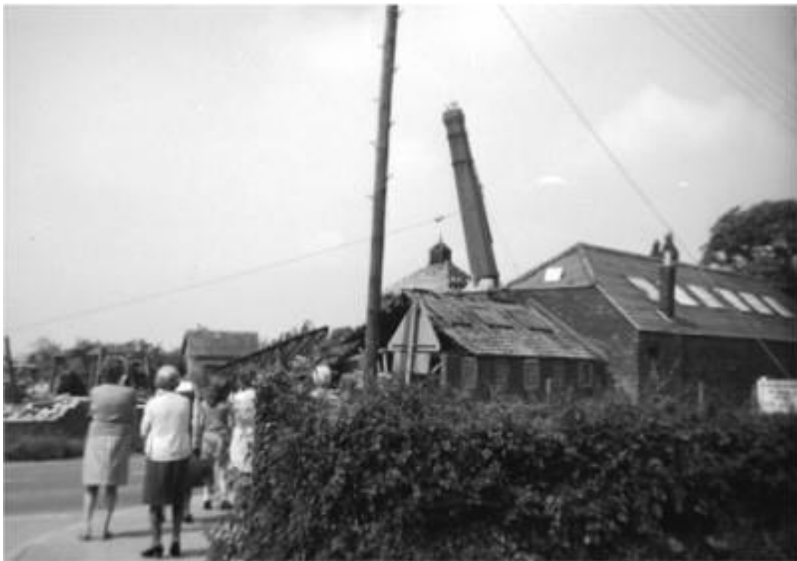
Demolition 1973 View from end of The Butts, looking across the main road. Smiths' shop and half the fitting shop already gone, and chimney on the way down!
